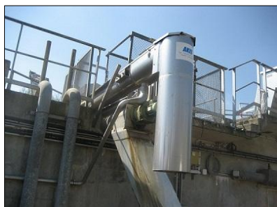
Spiral Press with trapdoor for back pressure
