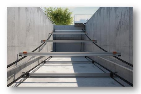
Scraper flights Fiberglass reinforced plastic and the sigma shaped profile of the flights makes it more corrosion resistant, rigid, strong and flexible to resist high sludge loads without compromising the safe operation. We define the suitable scraper profile based on tank dimensions and sludge load. The scrapers are equipped with skids and filler blocks for the strongest possible fixation of the chain's.
